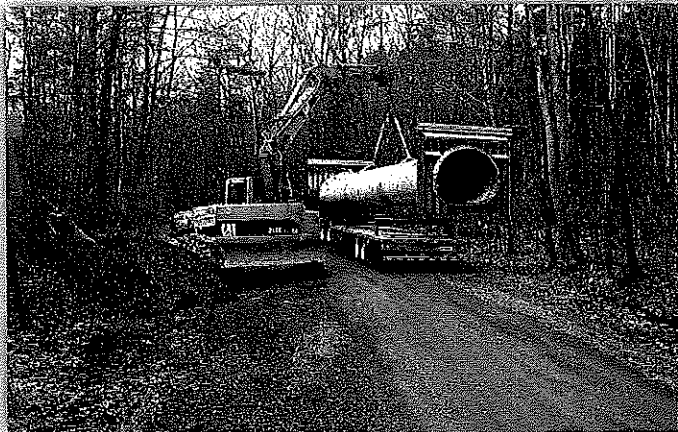
A new 6' oval pipe is lifted into place in Huntingdon County.
