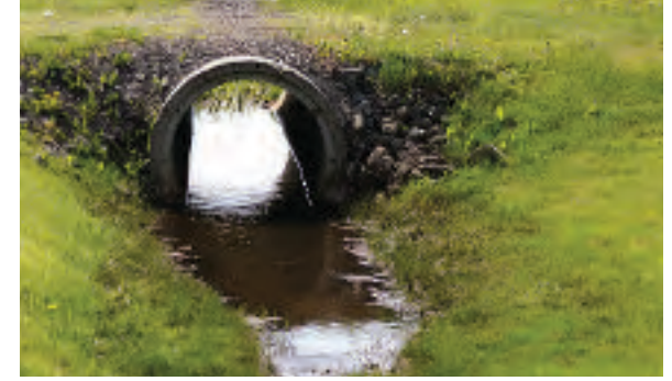
MINOR ROAD CROSSINGS
