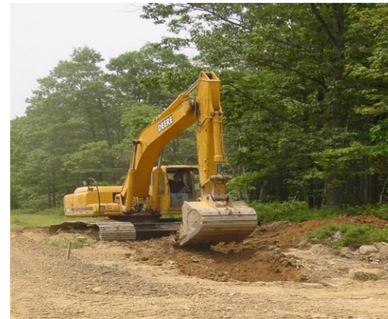
Earth disturbance can increase erosion and sedimentation and pollute surface water.
