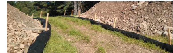
Compost filter sock prevents sediment from washing off the construction site.
