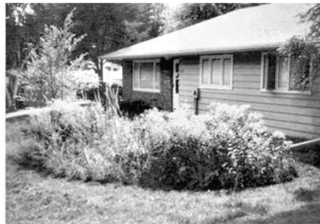
Rain gutters direct rooftop runoff to this attractive rain garden reducing stormwater problems for the homeowner and neighbors
