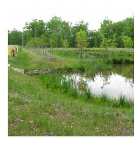
Detention BMPs, such as the detention basin pictured above, provide a delayed and controlled release of runoff. This helps to:
