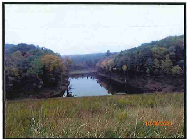
Leavitt Branch Dam
