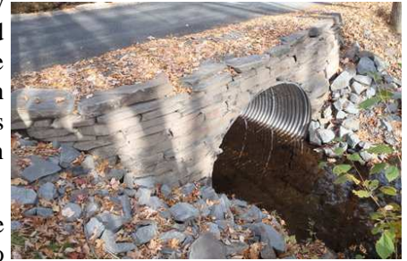
Overflow Stream Culvert Installed, Bluestone Boulevard, Westfall Township
