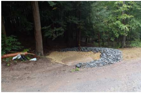
Mt. View Road Stilling Basin in Greene Township
