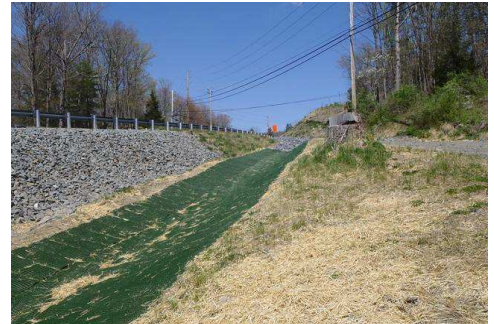
Pictured above in green is Turf Reinforcement Matting used for channel stabilization
