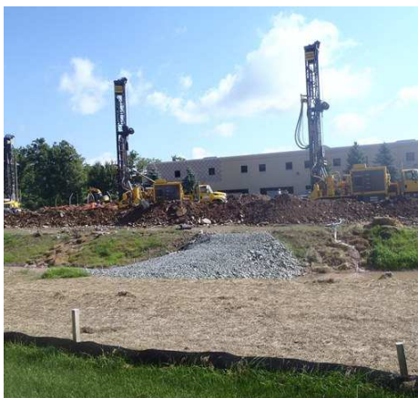
Pictured above: Geothermal wells being installed at the Wallenpaupack Area School District site
