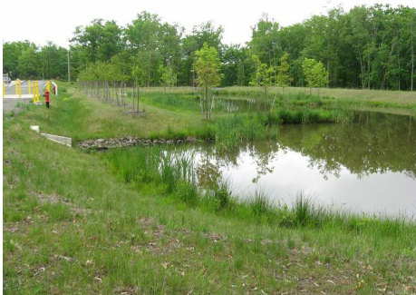
Pictured above is a stormwater detention basin
